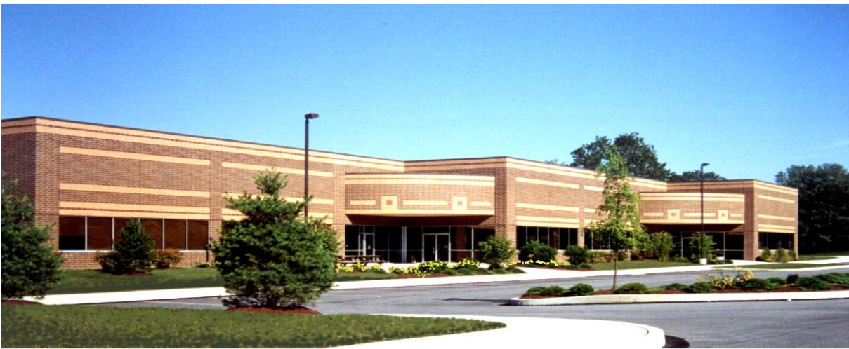
Clean Room R & D Facility, Exton, PA
